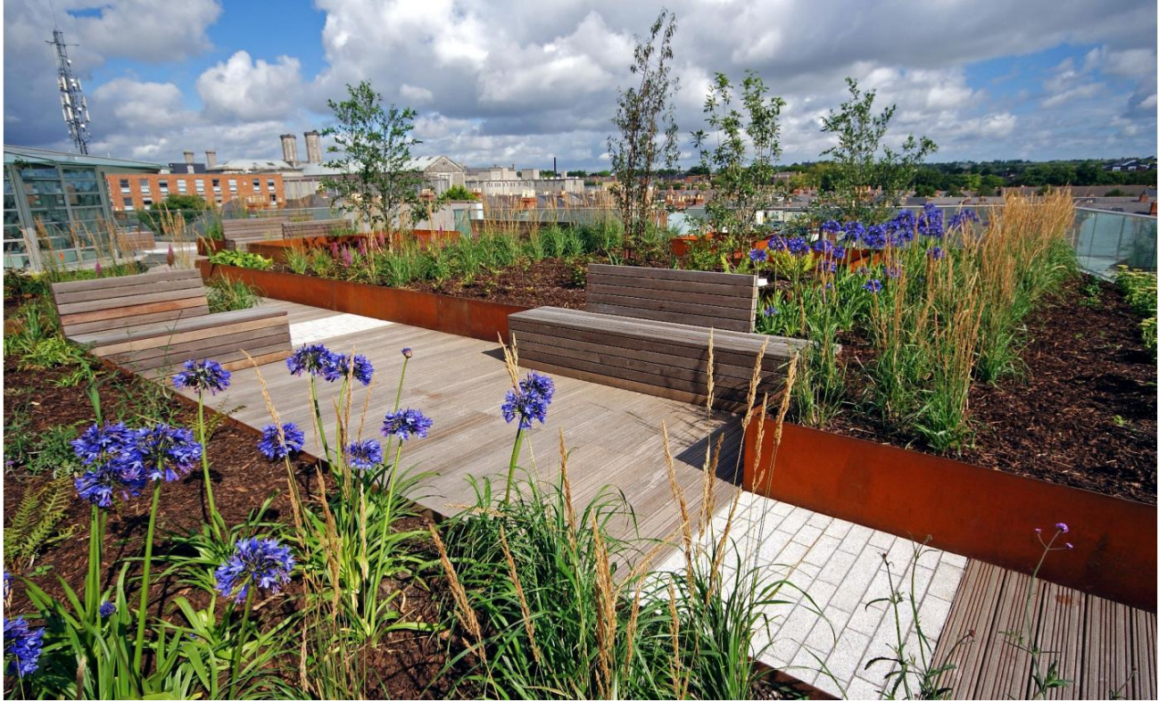
Above: view looking north across central seating area. Topsoil depths 300mm increasing to approx 600-800 mm depth provision at trees. Photo taken summer 2012, approx 4 months post completion.
